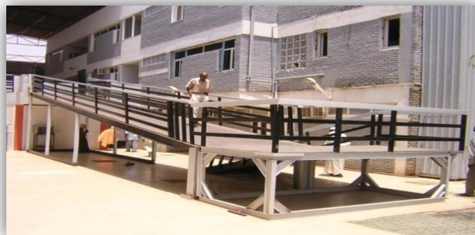
Figure 5-21 Ramp link between wards
