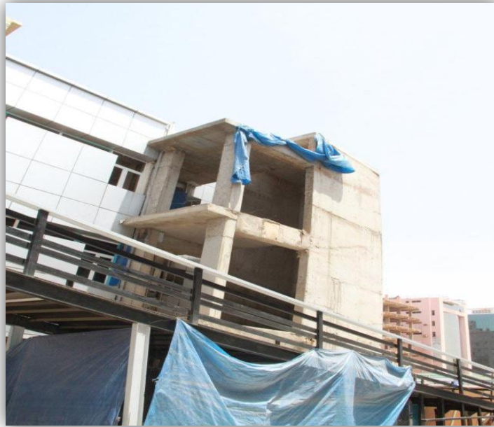
Figure 5-22 Lift under construction
