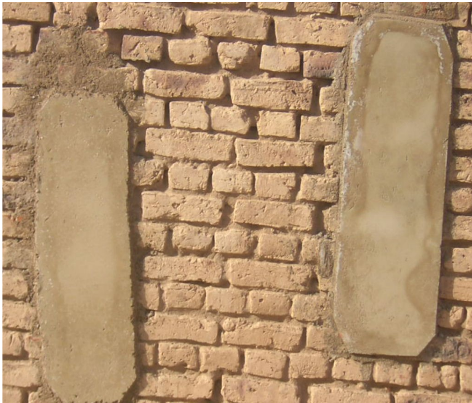
Plate C5: Wall plasters Strips (left: test sample, right: control sample)
