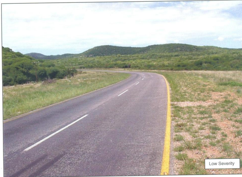
Photo 1: Rutting (Distress Type 15)
