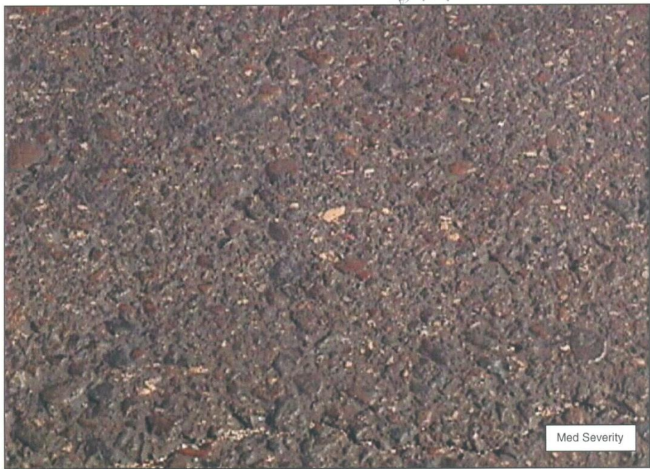
Photo 2: Polished Aggregate (Distress Type 12)
