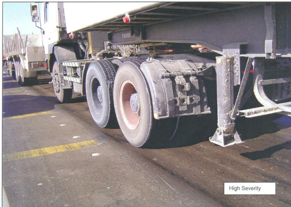
Photo 4: Rutting (Distress Type 15)
