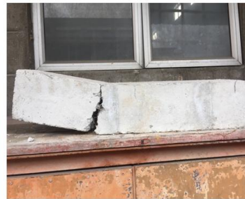
Prism failure (left view) – almost splitted into two sections
