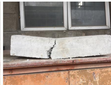
Prism failure (left view) – almost splitted into two sections
