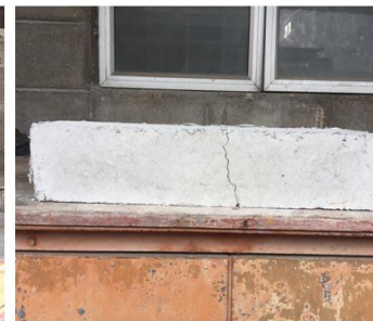
Prism failure (left view) – only cracks appeared
