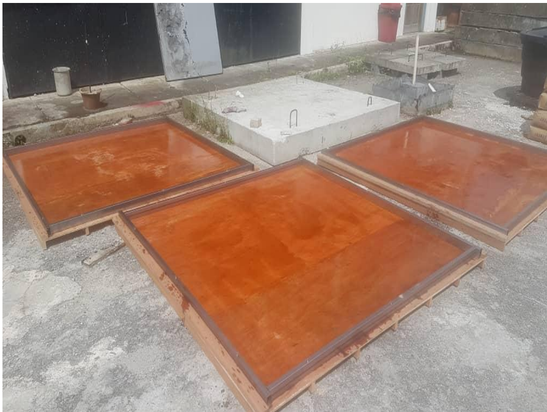
Figure 3.12 Manufacturing of Formworks and Casting Specimens
