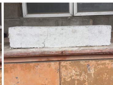
Prism failure (left view) – only cracks appeared
