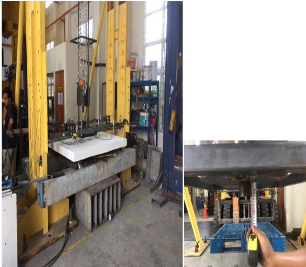
Figure 3.13 Typical Specimen Setup Before Testing
