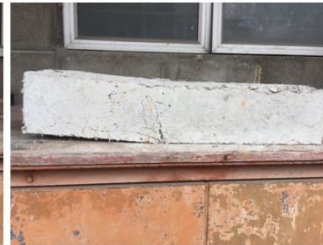
Prism failure (left view) – only cracks appeared
