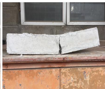
Prism failure (left view) – almost splitted into two sections
