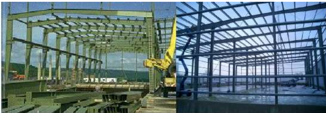
Figure 4.2: Industrial Hall using Steel Frame System.
