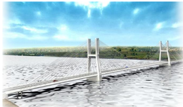
Figure 2: TUTI BAHARI cable stayed bridge
