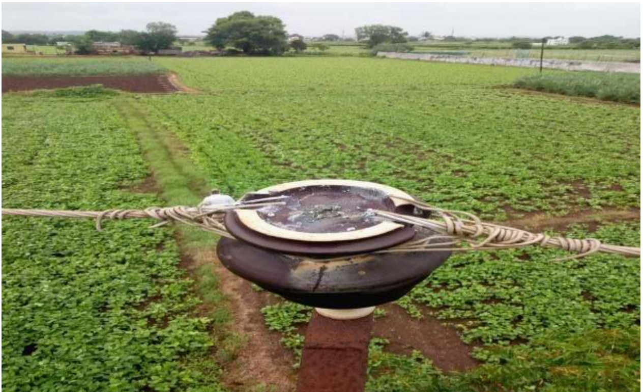
Figure 4.16: spindle insulator hidden conductor cutting
