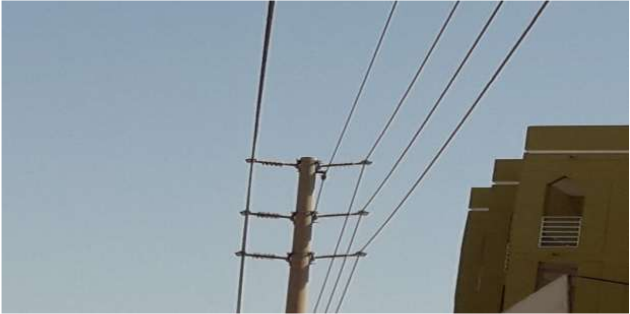
Figure 4.15: line post insulator configuration
