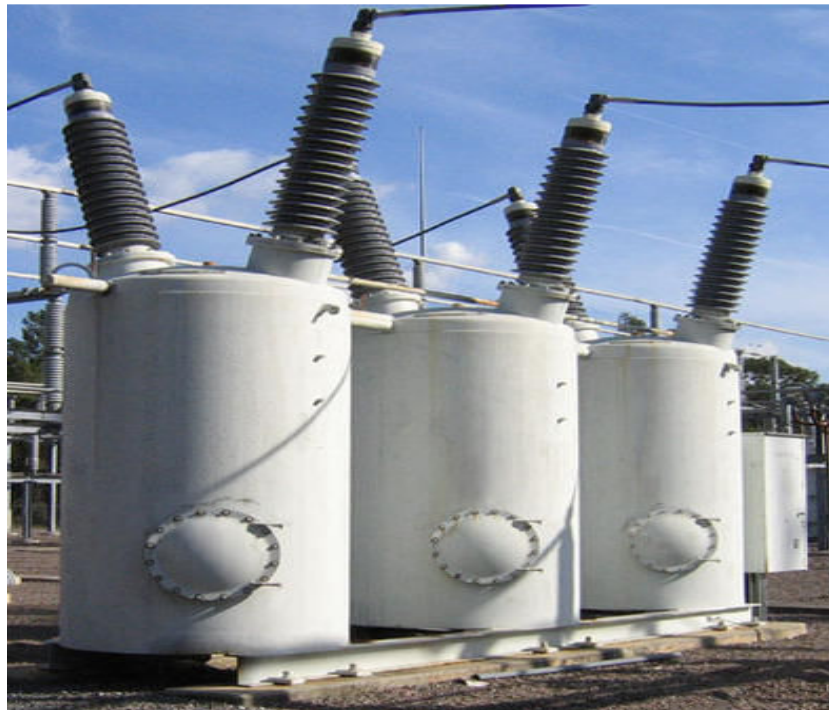
Figure 2.10: Minimum oil circuit-breaker
