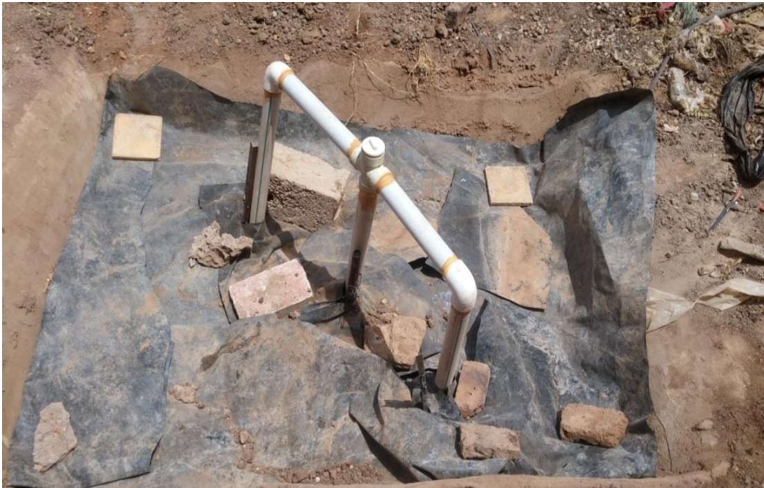
Fig (3.14): Geomembrane in final cover.
