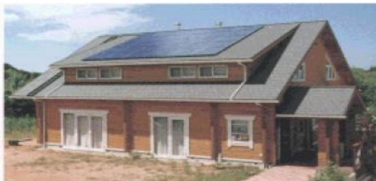
Solar Cell Capacity: 4.35 kW
