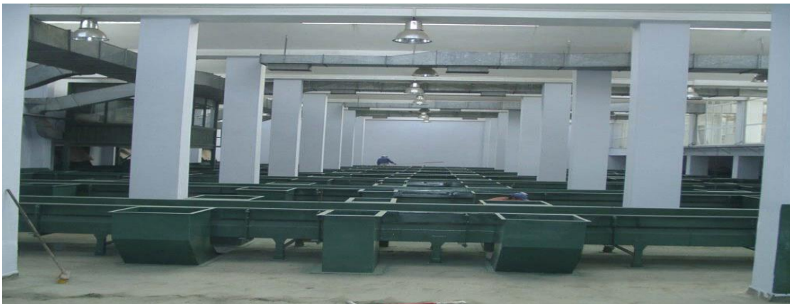
Fig (2.6) : Packaging Waste Separation Facility in Ankara, Turkey (KÖSE et al., 2007).
