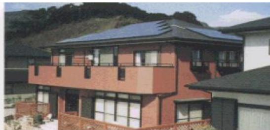
Solar Cell Capacity: 3.48 kW
