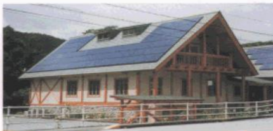
Solar Cell Capacity: 14.36kW
