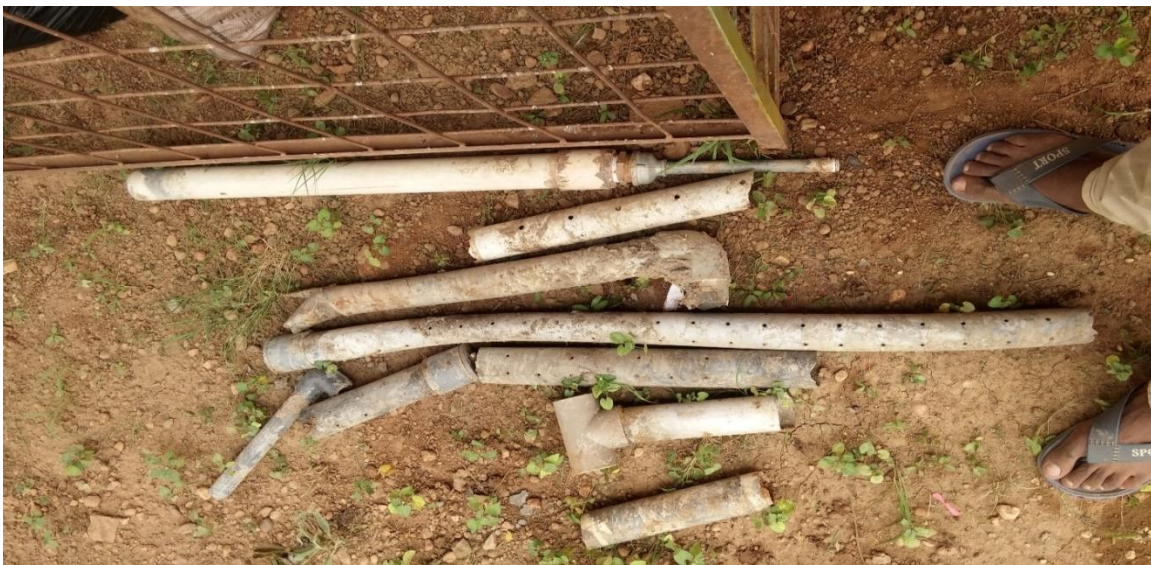
Fig (3.6): old gas extraction pipes.
