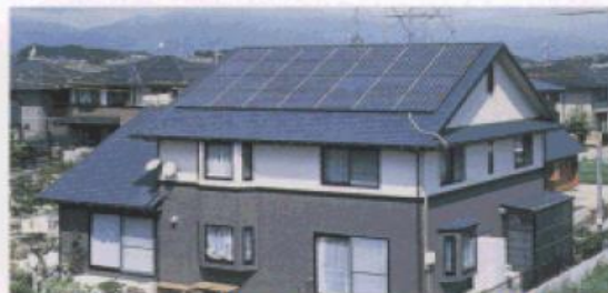
Solar Cell Capacity: 3.92kW
