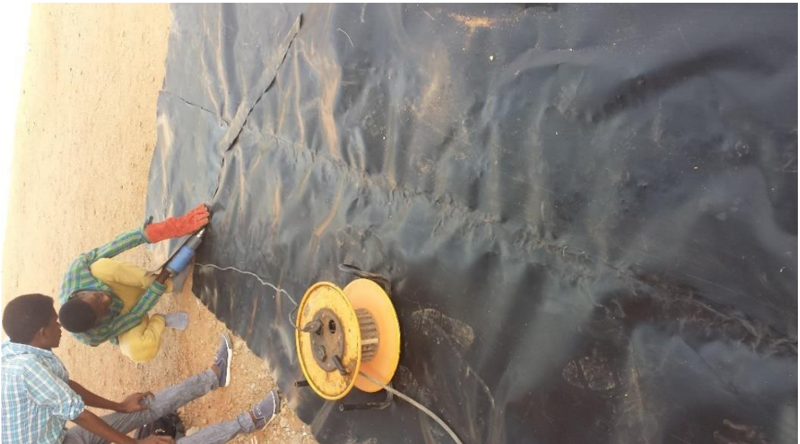
Welding of Geomembrane
