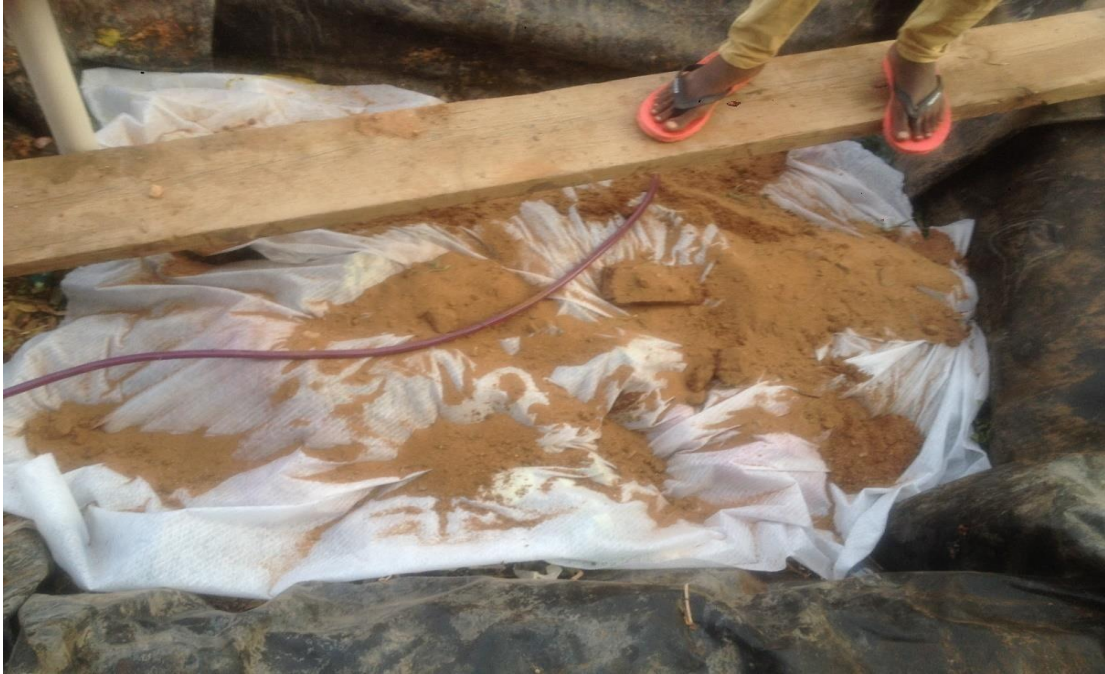
Fig (3.13): Geotextile in final cover.
