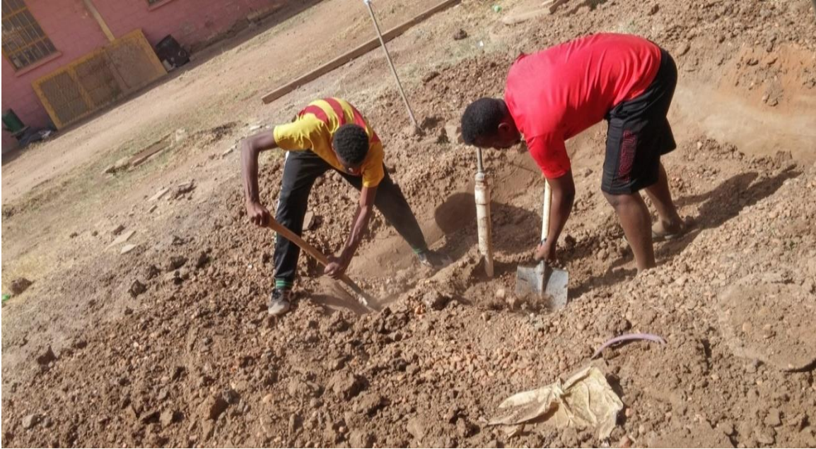
Removal of soil layer
