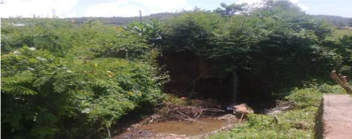
Figure 4.12 initially constructed one Rows of Pipe Culvert at Station 0+85
