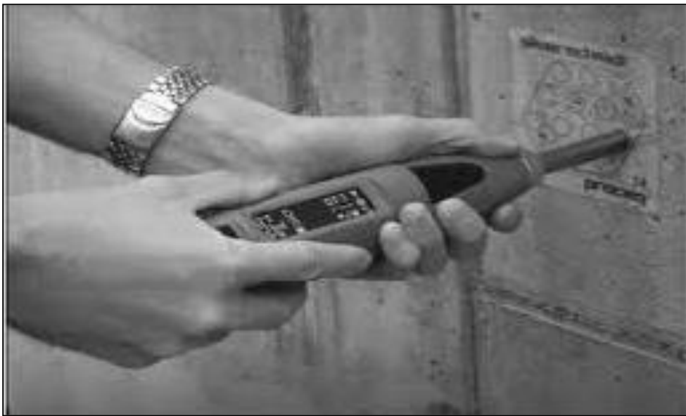
Fig.(2.1): NDT of concrete by Schmidt Rebound Hammer.
