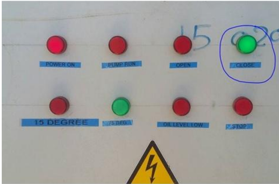
Figure 4.15: Hydraulic valve fully close position
