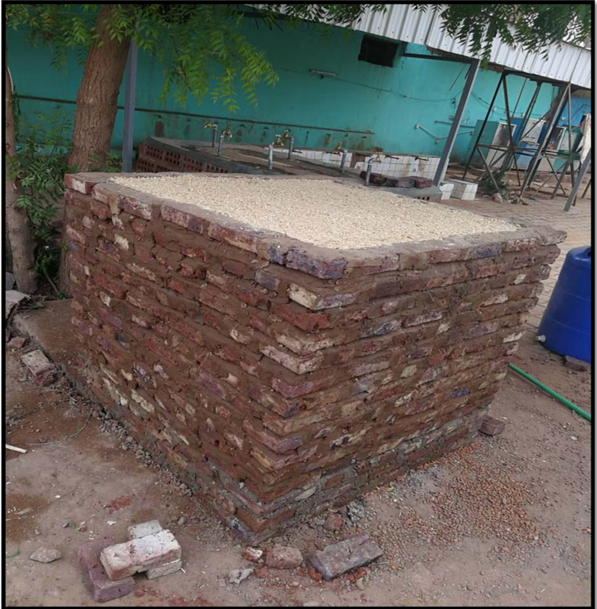
Figure(3.3): the layer of insulation on the base.
