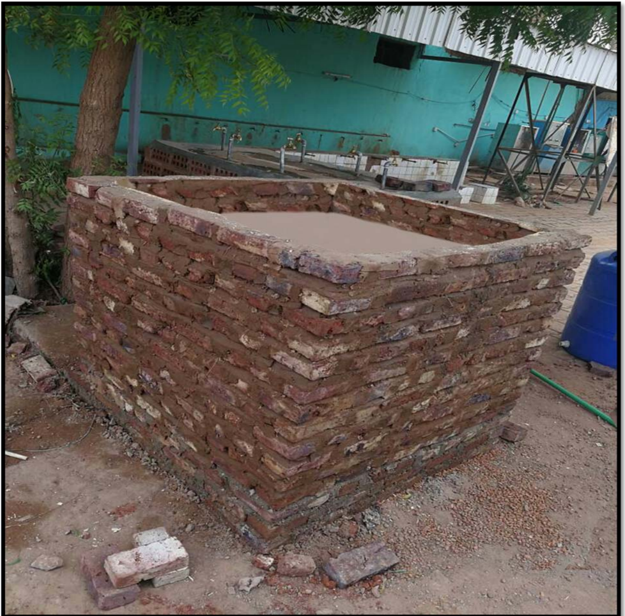
Figure(3.2): the base of thermal storage.
