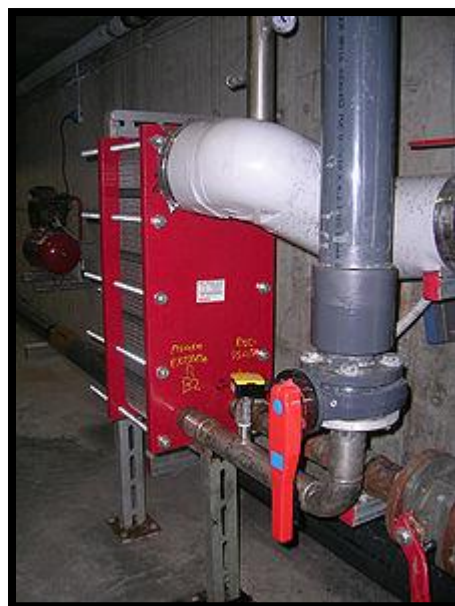
Fig3.22A single plate heat exchanger.
