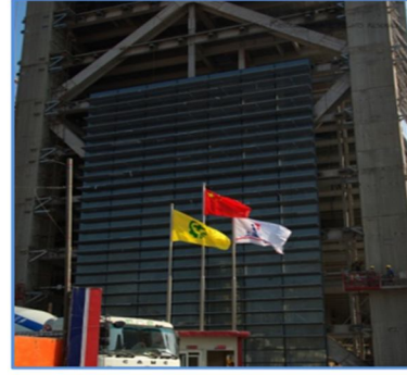
PVs solar shaded on the E&W facade
