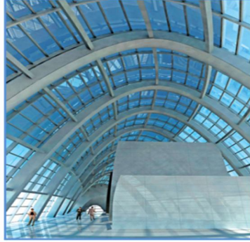
Top Of The Tower Integrated Photovoltaic'
