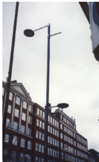
Figure 3.3 Piggyback lighting to illuminate footway as well as carriageway
