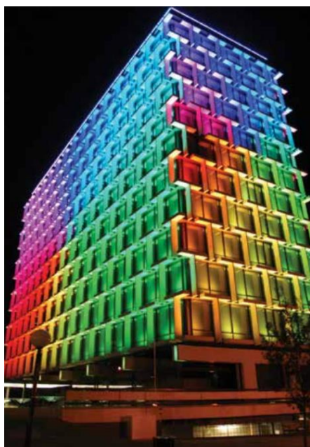
Figure 3.11 building lighting Source: exterior building lighting
