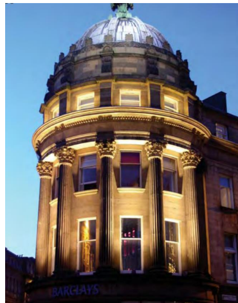
Figure 3.19 lighting selected feature Source: external lighting for historic buildings
