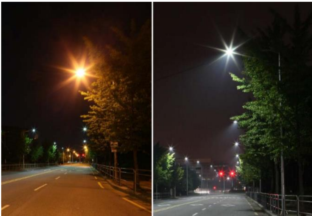
Figure 3.10 comparison between HPSV (left) and LED (right) Source: LED road lighting design manual
