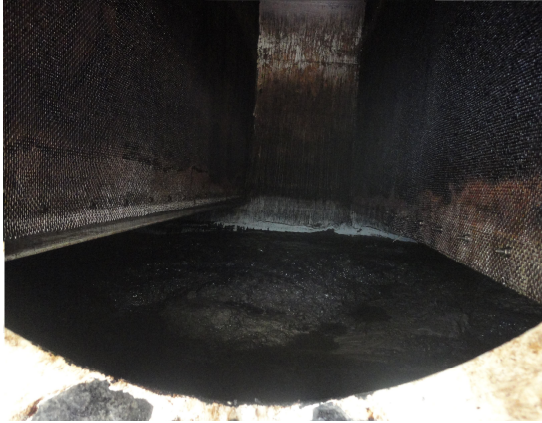
Figure 2-15: Sludge inside heater treater
