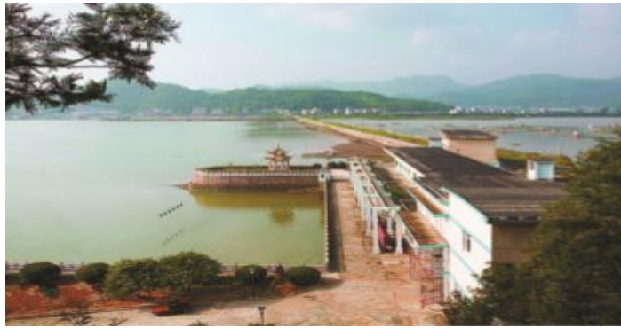
Figure 3.5 Jiangxia tidal Power Plant
