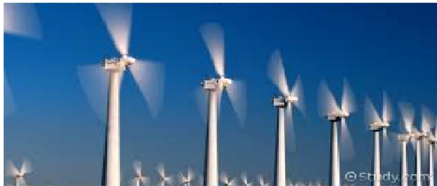
Figure 2.2: wind turbine farm
