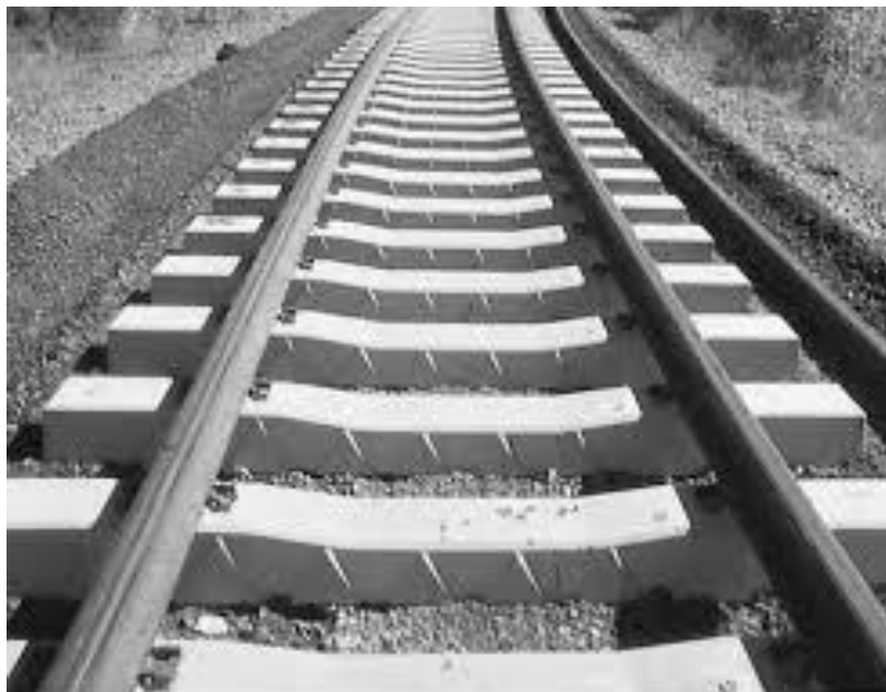
Fig (3/10) Concrete Ties - Photo by Kevin Keefe
