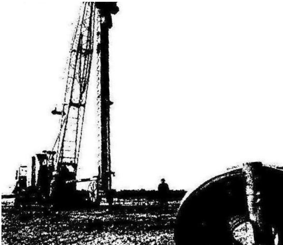
Fig (3/3) Vertical drainage installation
