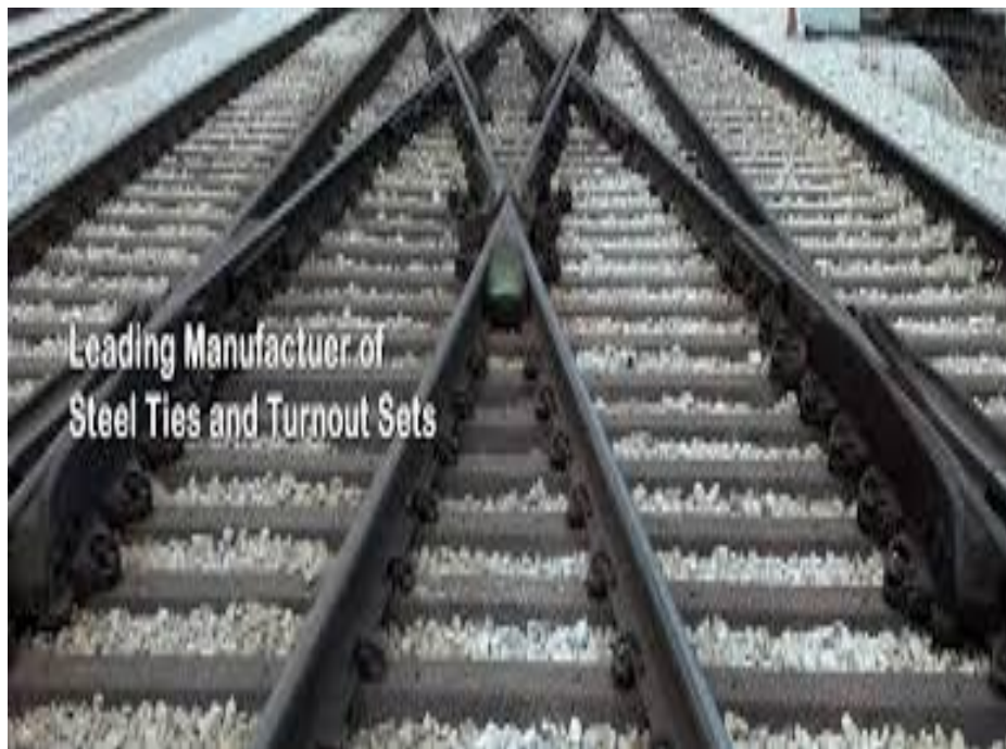
Fig. (3/11) Steel Ties
