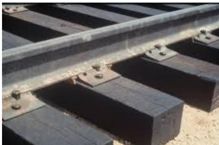
Fig (3/7) Hardwood Track Ties - Photo by J.E.Riely
