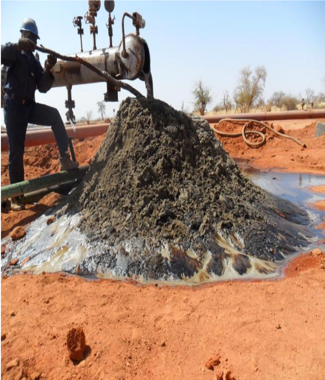
Figure 4.19 Sand Cleaning of FNE OGM-1
