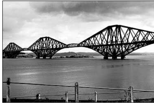
Fig. (2.4) :Truss Bridge.
