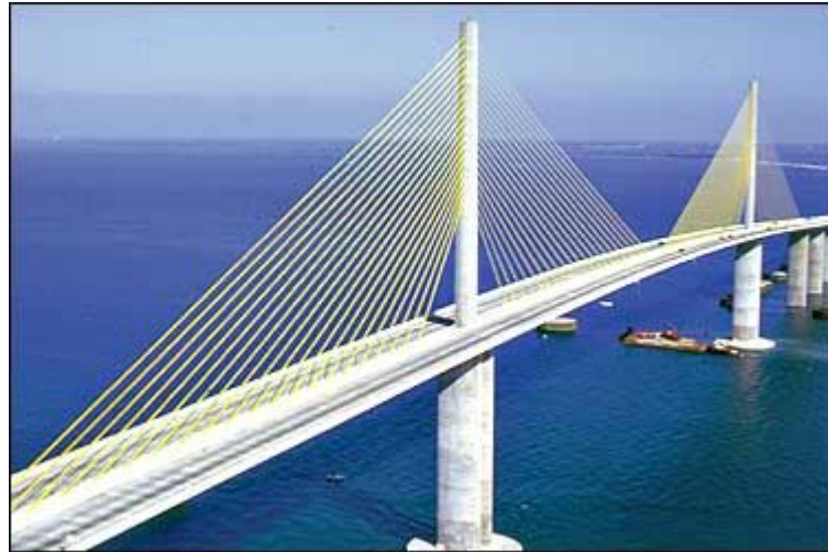
Fig. (2.6): Cable-stayed Bridge.
