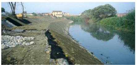
Fig. (5.19): Guide Bank Failure
