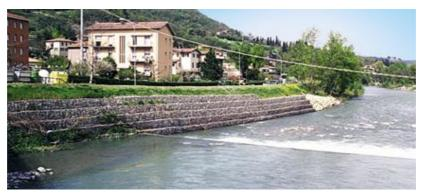
Figure (517): Typical Guide Bank Gabion Walls
