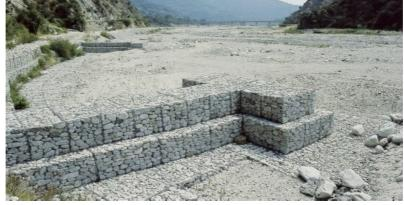
Fig.(5.18): Typical Gabion Groins Construction
