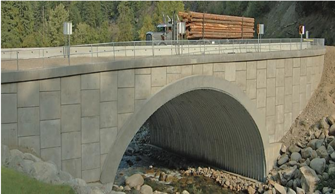
Figure 2.25. Steel structural plate Arch culvert. [11]
