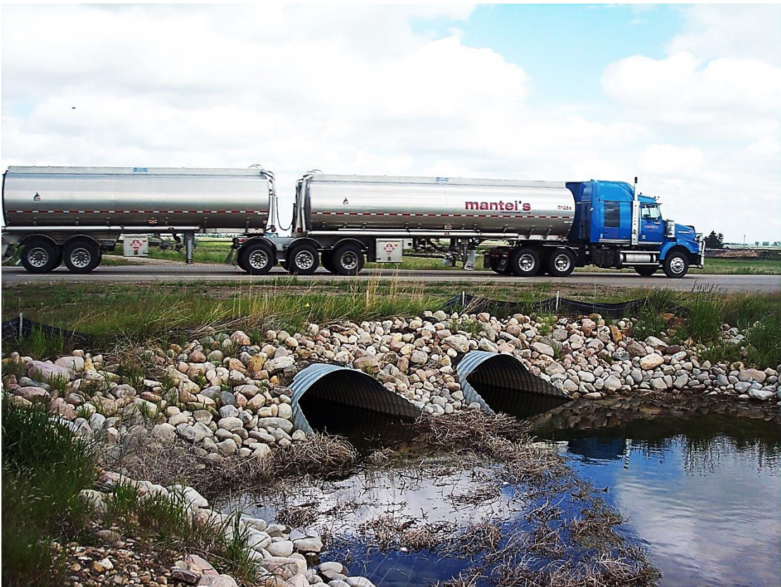
Figure 2.24. Corrugated steel pipe culverts. [10]
